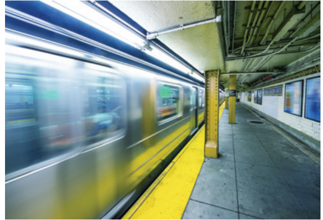
Figure 6 – Train platform and trainway
